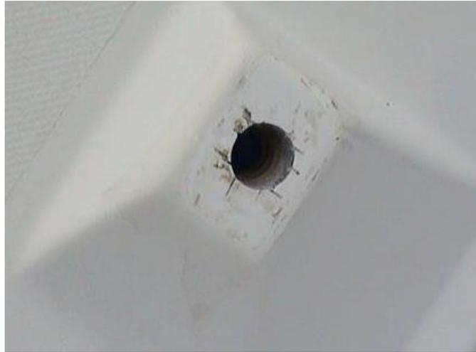
This is a typical hole after it had been drilled. The scoring lines are from a previous attempt with the Dremel to cut square chunks out. I realized right away that this was not going to be the way to do it.
