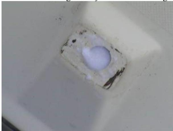
I filled each hole with epoxy, packing it in until it was over the top of the hole. I then put 3M long term masking tape over each one to smooth out the top surface and further pack the epoxy in. It was also looking like it was going to rain (it did – buckets), so the tape helped keep the water out while the epoxy cured. The temperature was in the low 50's so I left everything to cure for a week.
